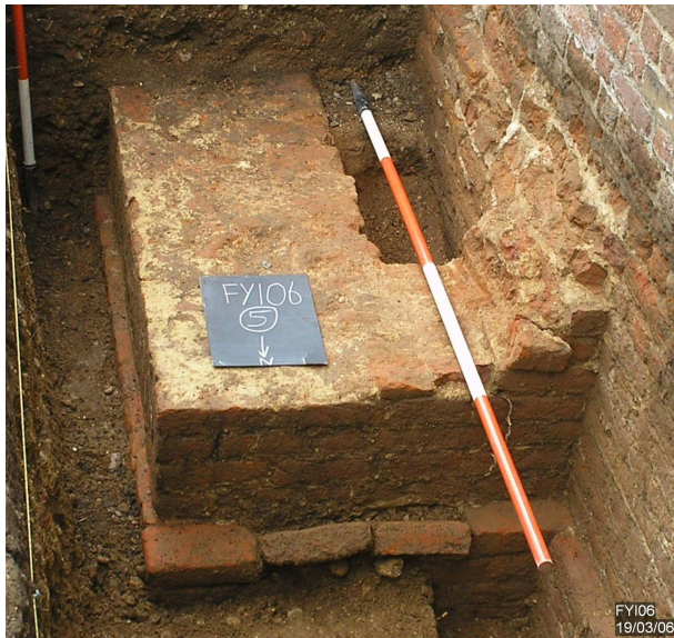
Foundation of bay window, Forty Hall (see page 7)
